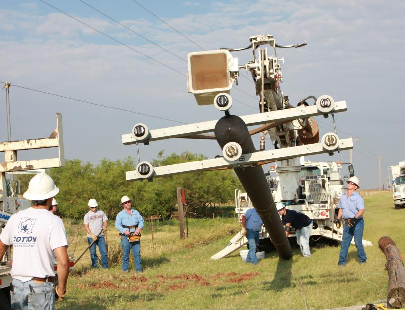
Our sand-hardened Ameron uPole utility pole is manufactured using Fiberglass Reinforced Plastic (FRP) materials. This series of distribution poles was developed in order to provide customers with a long-lasting, cost-effective alternative to distribution poles made from wood, steel and pre-stressed concrete. Since it was introduced to the utility market in 2008 it has been accepted on standards at over 100 IOUs, municipalities and electric cooperatives and the list is growing.
